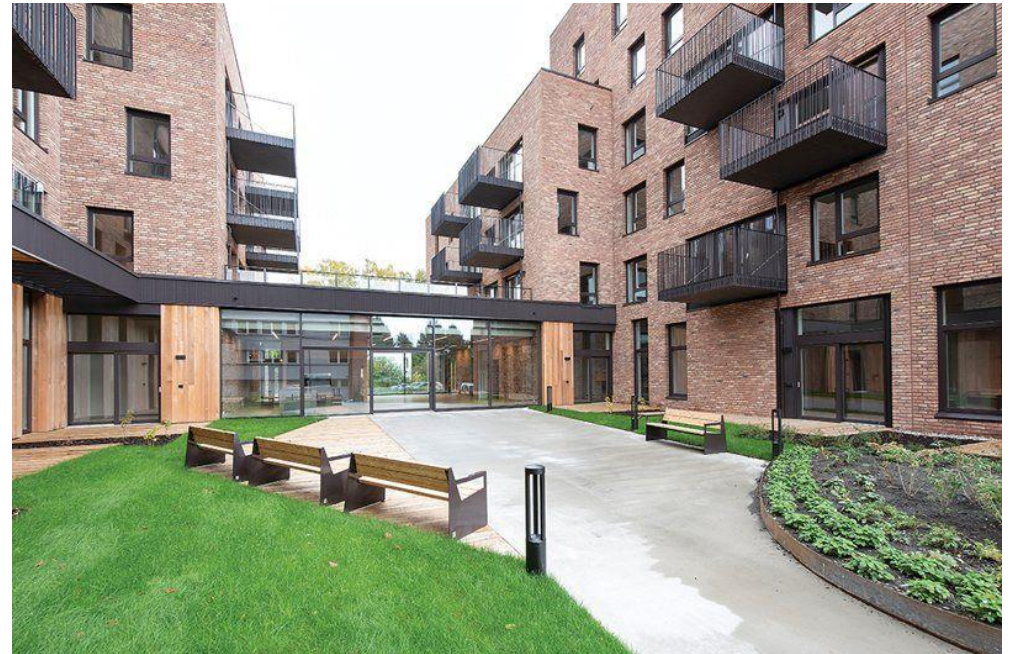
Reference project, Diakonveien Omsorg, masonry and plastering work
